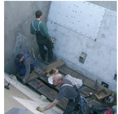
Stud-welding process: lining a hopper
